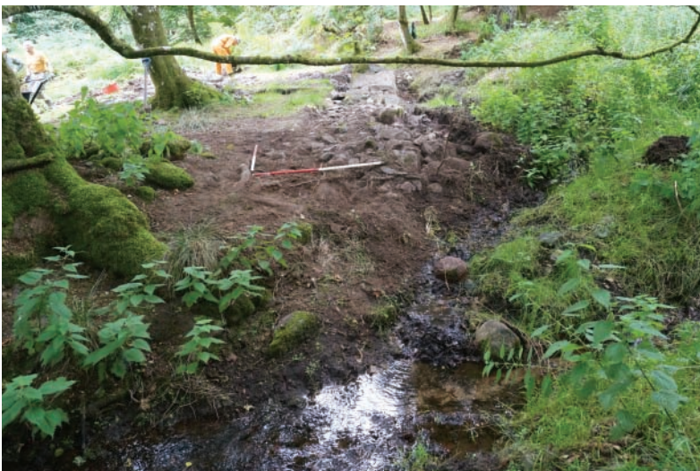
Photo 3. Water channel possibly cutting wall [A].
